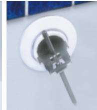
4-5. Install/remove universal wall fittings. Place hex bar in hole for more turning and torque.
